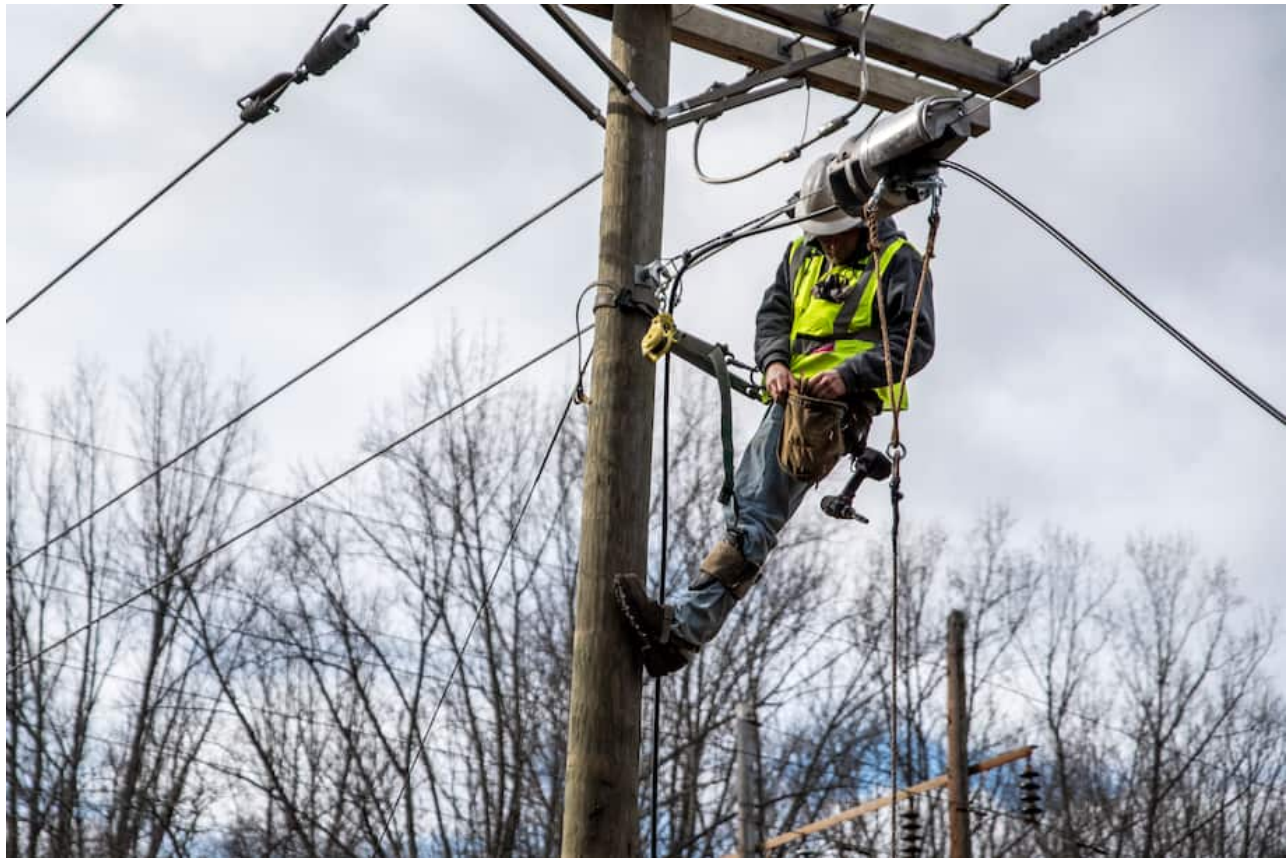
Crews work to hang fiber-optic cable in Amherst, Va. (Kendall Warner/AP)
